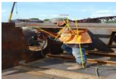
**Figure 2. Standing Work Posture in Welding**
